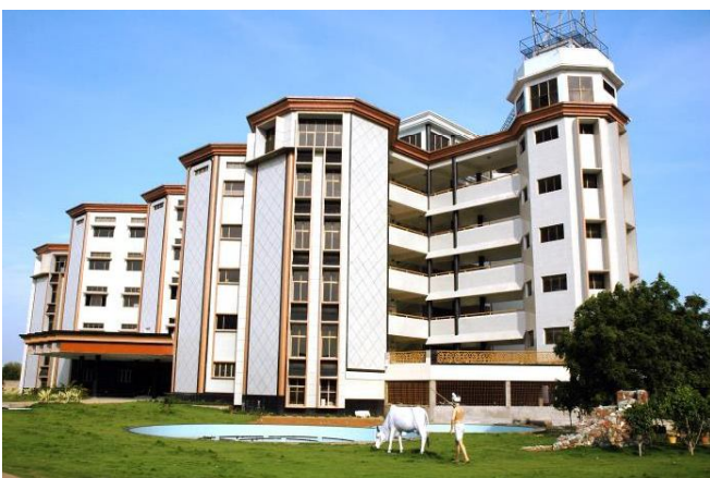
GENERAL ENGINEERING BLOCK
