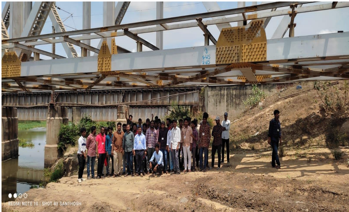
A field visit to steel truss and girder bridges near vedullapalli, Bapatla on 27-05-2022
