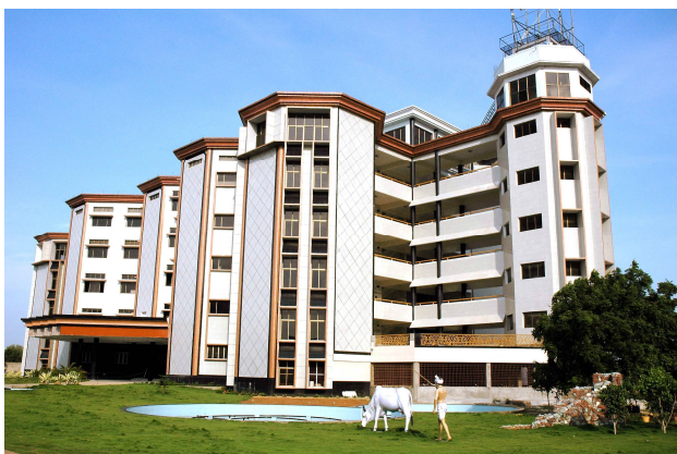
GENERAL ENGINEERING BLOCK
